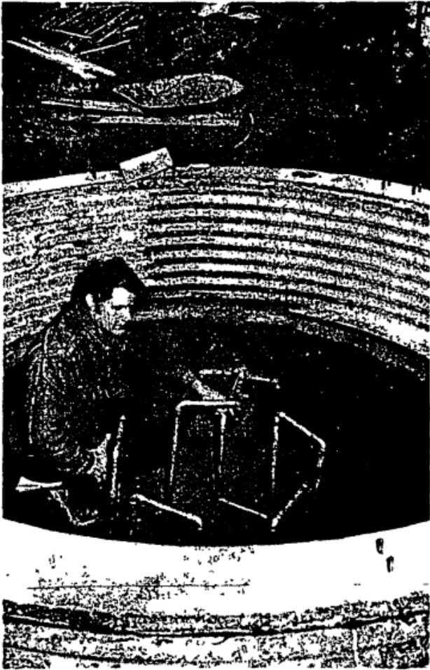
HEATING SYSTEM —Stanley Meyer begins installation of the heat exchanger in the storage cavity of the solar thermal electric power generation system he is building on Marlane Drive. A translucent silo-lens structure will be constructed above the storage cavity to collect sun rays.
