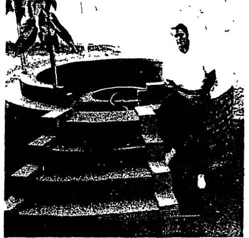
STANLEY MEYER poses on the base of the solar energy device he is building just outside Grove City. The base will house two heat energy storage tanks as well as a steam-driven engine. The frame of the device will hold up a silo-shaped collection of lenses which will focus the sun's rays into the storage tanks, Meyer says.
