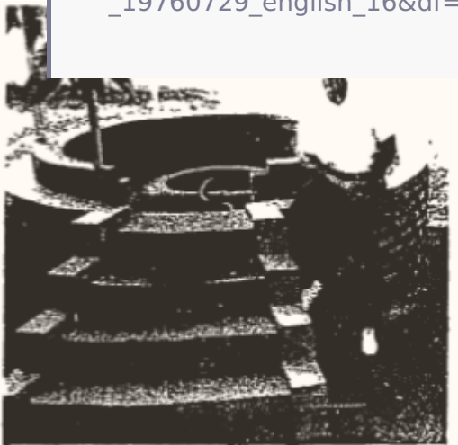
STANLEY MEYER poses on the base of the solar energy device he is building just outside Grove City. The base will house two heat energy storage tanks as well as a steam-driven engine. The frame of the device will hold up a sloped collection of lenses which will focus the sun's rays into the storage tanks, Meyer says.
