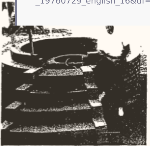
STANLEY MEYER poses on the base of the solar energy device he is building just outside Grove City. The base will house two heat energy storage tanks as well as a steam-driven engine. The frame of the device will hold up a sloped collection of lenses which will focus the sun's rays into the storage tanks, Meyer says.
